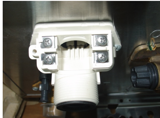
Figure 3. External connection to terminal block
